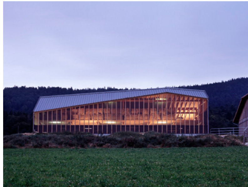
Local Architecture, stalla a Lignières, 2004
